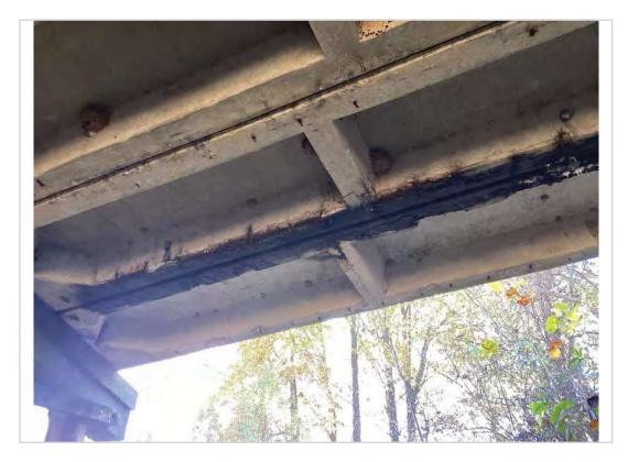
Span 1 PCCS 'H' spalling to steel with section loss
