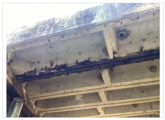
Span 1 PCCS 'I' spalling to steel with section loss
