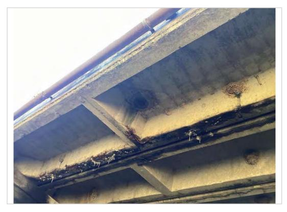
Span 2 PCCS 'A' spalling to steel with section loss
